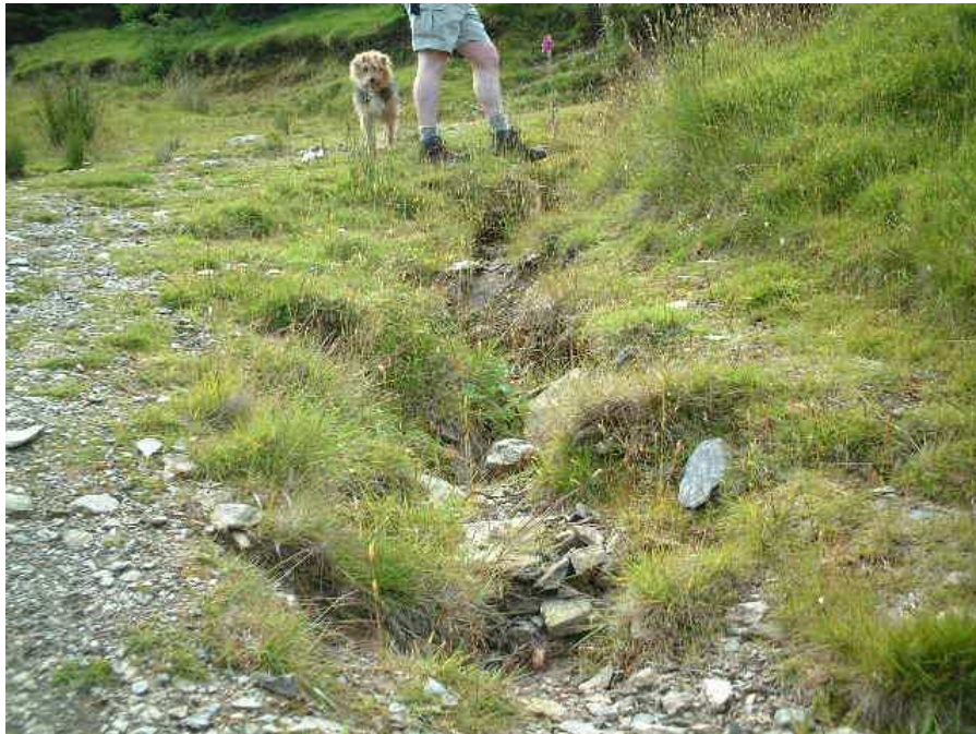
pic45 shows deep gully on the forest track; just above this there is a badly eroded bank at the next crossing of the track
