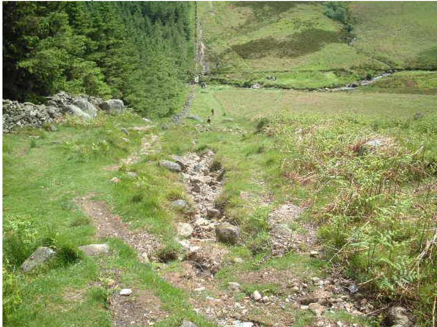
pic1 looking back down, shows the path; walkers turning into the forest to follow the Wicklow Way below; note water damage in the middle of the path
